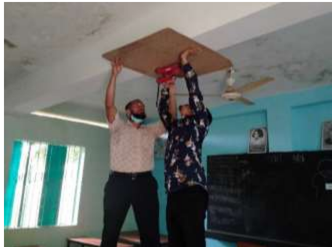
Figure 5.2: Ferro-scanning of a beam
