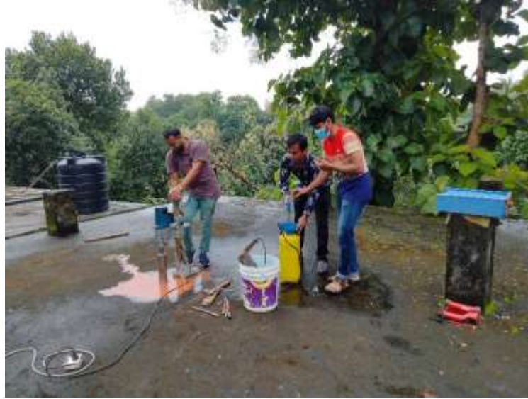
Figure 5.1: Core extraction from roof slab
