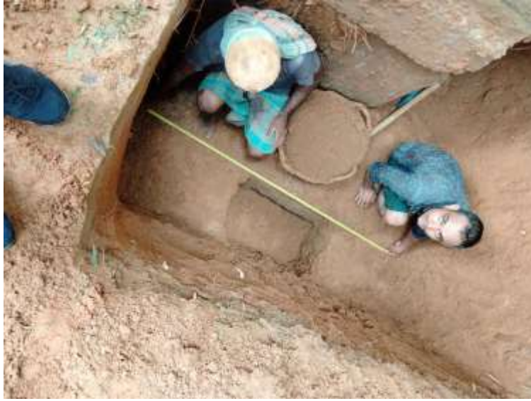
Figure 5.3: Footing excavation
