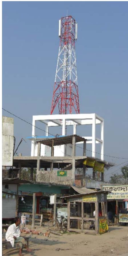
Figure 18: Typical Mobile Telecommunications Tower
