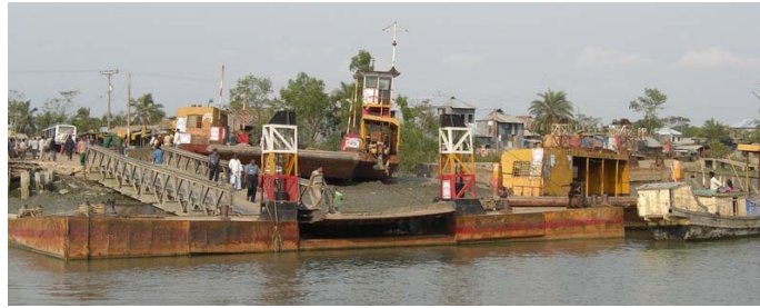
Figure 16: Ferry Pontoon with Stranded Ferry
