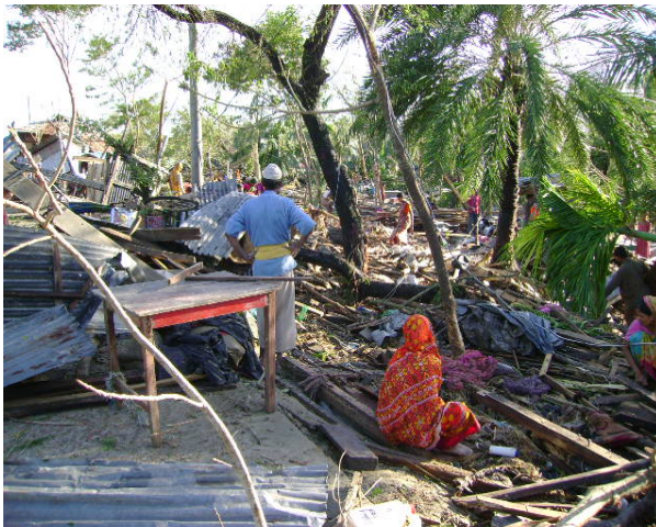
Figure 1: Destroyed Houses at the Coast of Bangladesh
